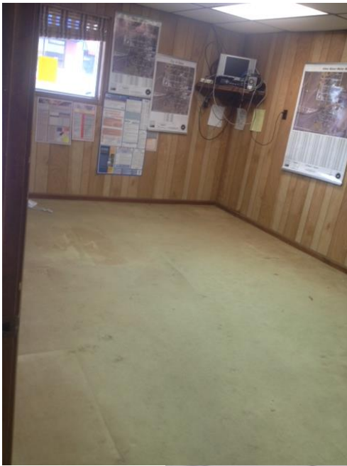
Office before new floor
